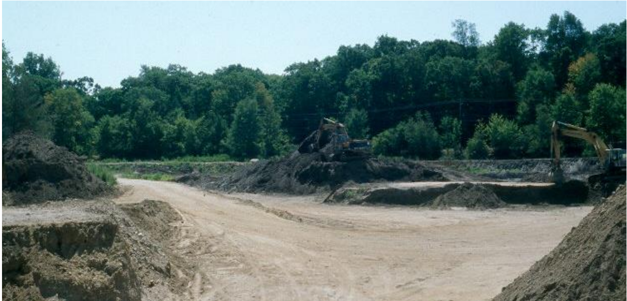
Figure 12. Dry dredging a small lake in Guilford, Connecticut.
